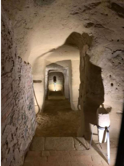
Led interno Ipogeo
